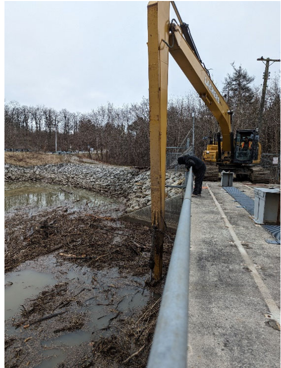
Many large logs and trees were wedged broadside along the face of the spillway which prevented the natural clearing of the debris during the high flows.
