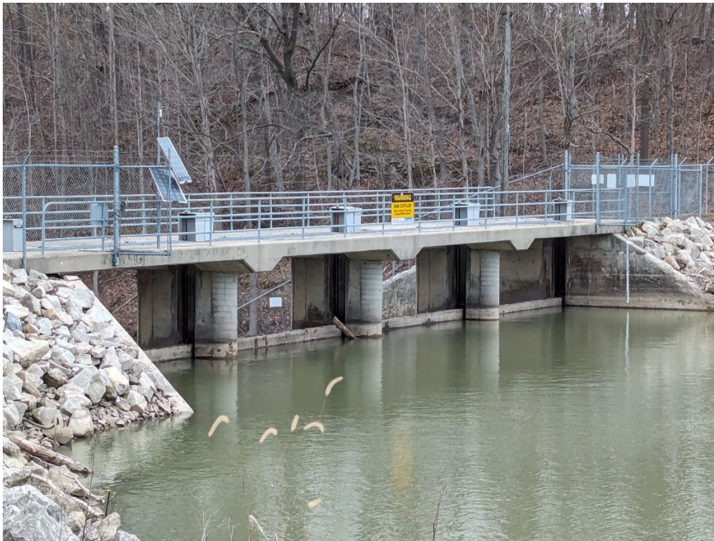
Stop logs back in position, March 19, 2024.
