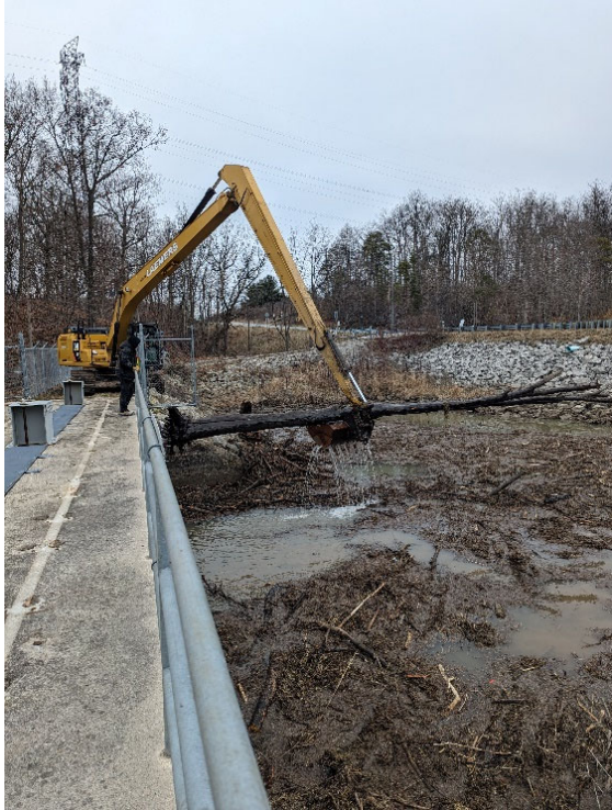
Many large logs and trees were wedged broadside along the face of the spillway which prevented the natural clearing of the debris during the high flows.
