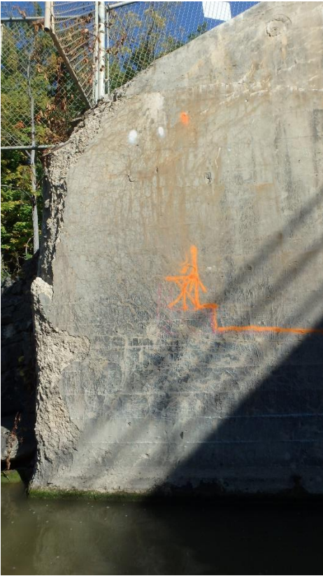
4. Corner of Downstream Retaining Wall at Wingwall
