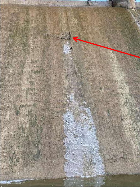
5. Spalling and Joint on Spillway Face – December 14, 2022
