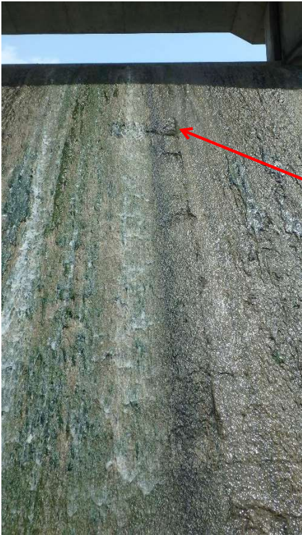
6. Spalling and Joint on Spillway Face – June 8 th , 2023 - No Change Observed
