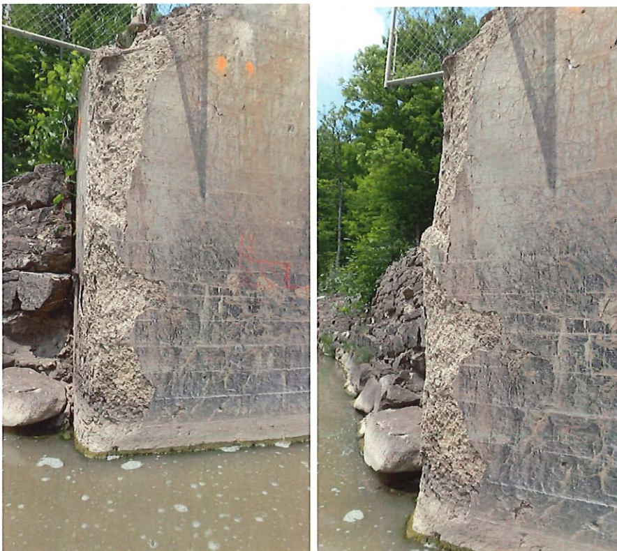
4. Corner of Downstream Retaining Wall at Wingwall
