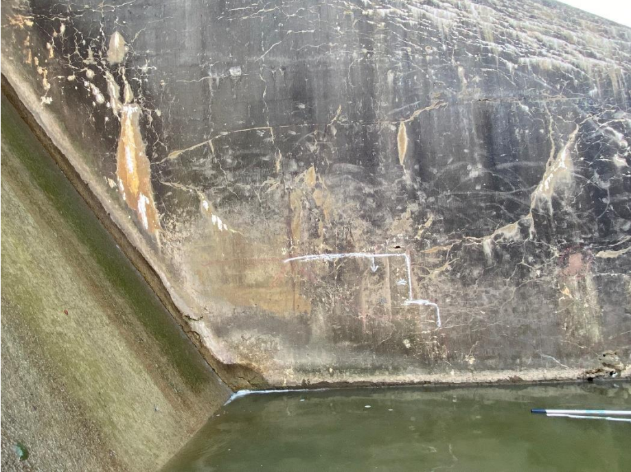
1. South Downstream Wingwall
